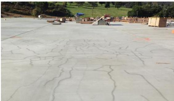
Typical roof deck shrinkage cracking (without the use of PREVent-C).
