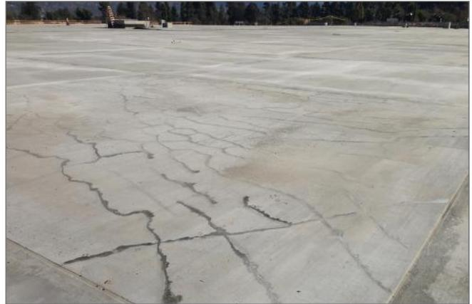
Typical roof deck slab showing extensive full-depth shrinkage cracks. These cracks are shown after epoxy injection repair and skim coating. Other minor cracking occurred but is not visible.
