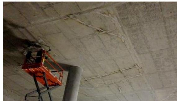
Repair of full-depth shrinkage cracking on the underside of the roof deck.
