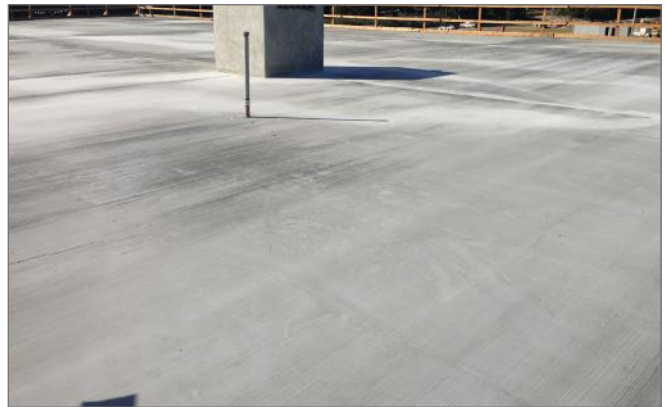
Test roof slab with 5.0% PREVent-C (above) shows no cracking needing repair.
